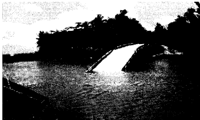
(b) Loss of support due to liquefaction, Rio Viscaya bridge, Costa Rica earthquake 1990
